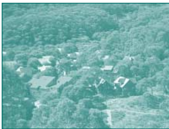
Photograph 1.1 Some past planning practices have provided little real protection to life and property in the event of a severe bushfire.
