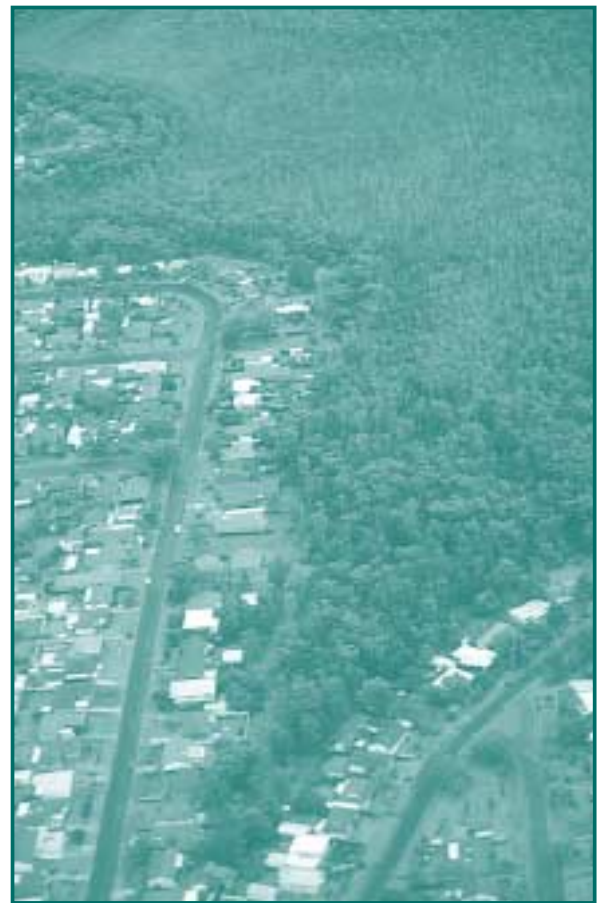
Photograph 1.2 Lack of separation places many properties in peril during a bushfire event. Fire fighters are not provided with adequate access to the hazard/development interface.
